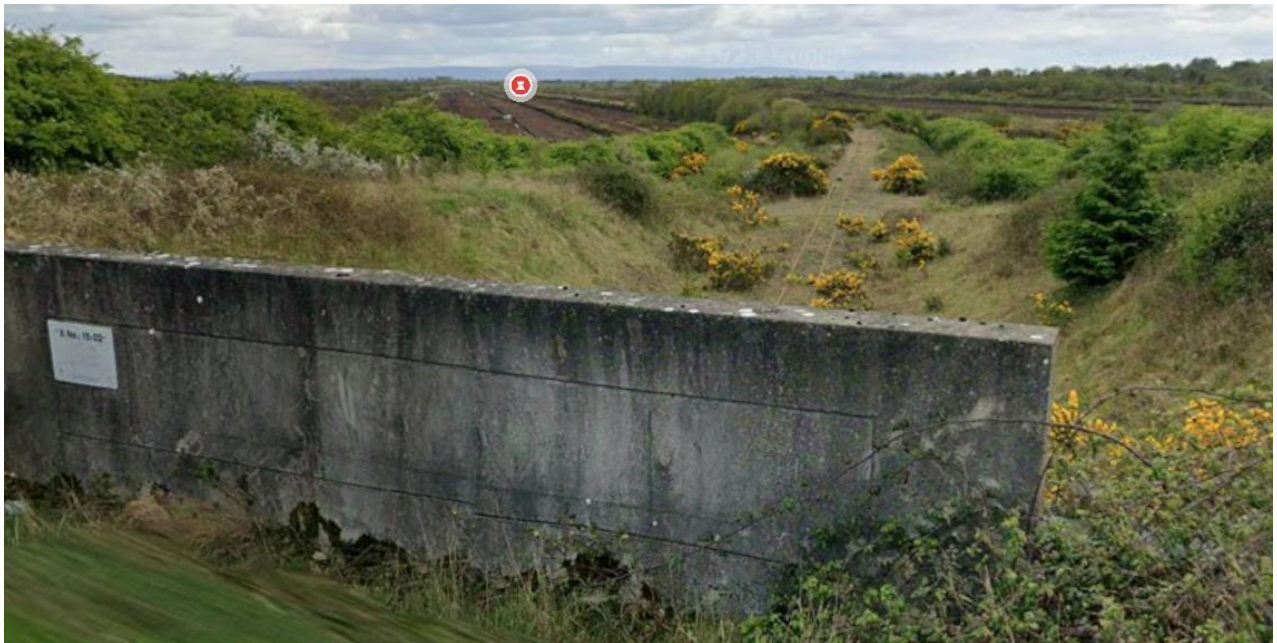
Image 9 - railway line between the two bogs
